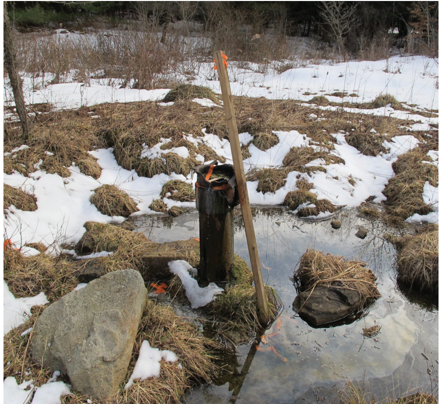
Image 18: Abandoned gas wells leak methane and other GHGs to the atmosphere and a program to identify and plug them with resulting offsets is being developed. Credit: Susan Phillips / StateImpact Pennsylvania
